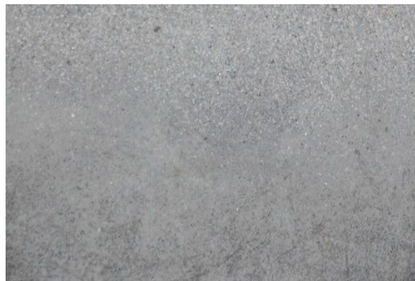
Clean Floor after Shot Blasting
